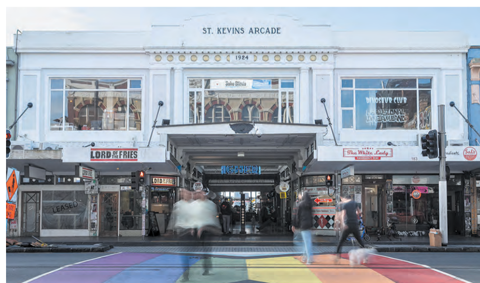
St Kevins Arcade on Karangahape Road.
